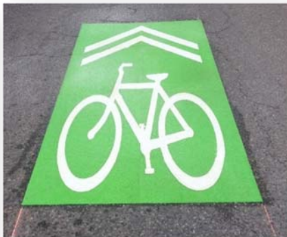
Figure 5 Sharrow on Green 1 Rectangle Pavement Marking
