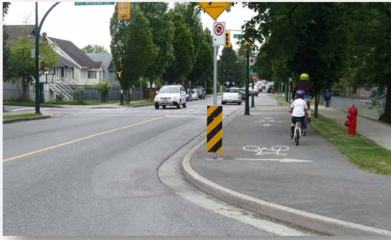
Figure 22 Example of an Off-Street Two-Way Cycle Track
