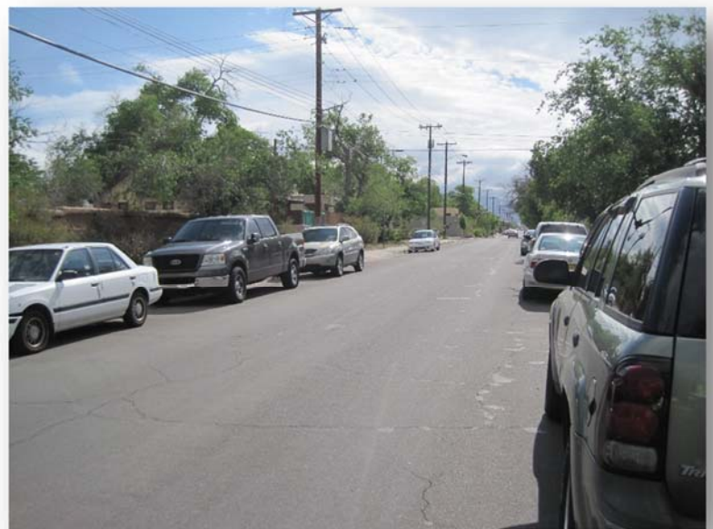
Figure 17 Existing Conditions on Silver between Girard and Tulane
